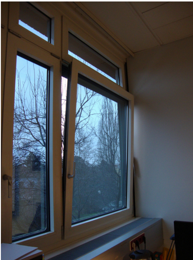
FIG 1 A bottom-hung window is a bottom-pivoting window that opens by tilting vertically, typically inside. It is also called a 'hopper window.'
